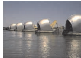
Figure 14: The Thames Barrier.
